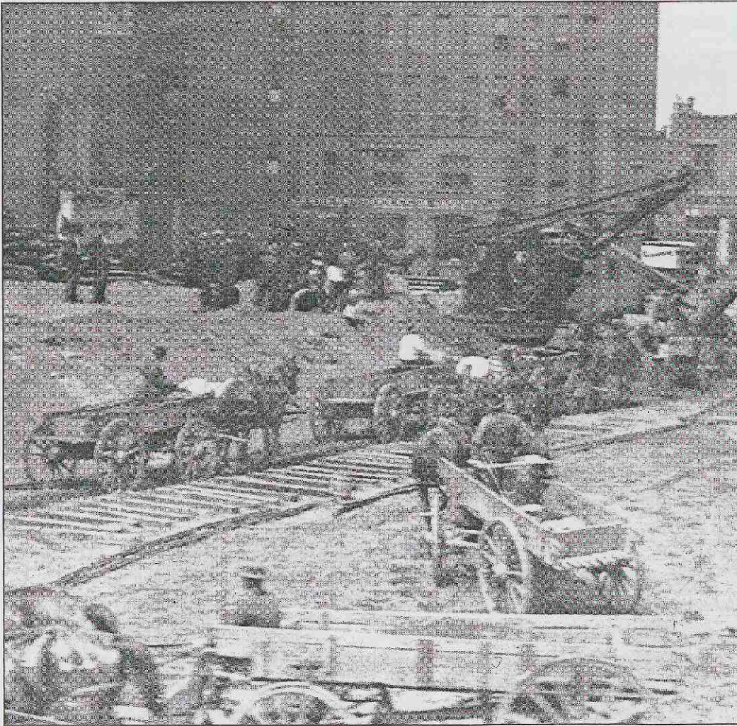
Fig 2: Horses at a Cleveland, Ohio, worksite, 1898.
