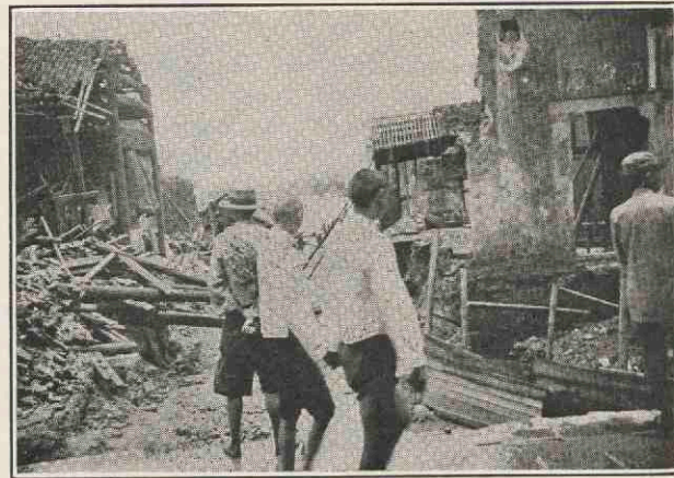
CHINESE HOMES IN CHANGTEH DEMOLISHED BY FLOODS
