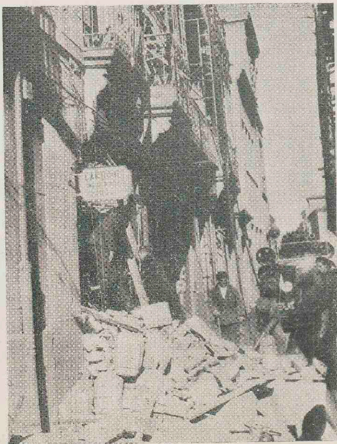
Damage the raid did in the Calle de Perez Pujol.
